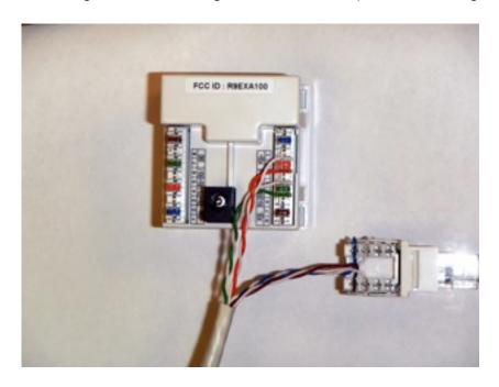
Using a Cat5 cable we are able to provide both power and 10 base networking to the WAP while at the same time using the spare 4 conductors to supply 2 analog lines.
