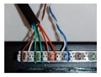
The image above shows the Green / Light Green / Orange / Light Orange used to supply both POE and data to the EXA100 WAP.
